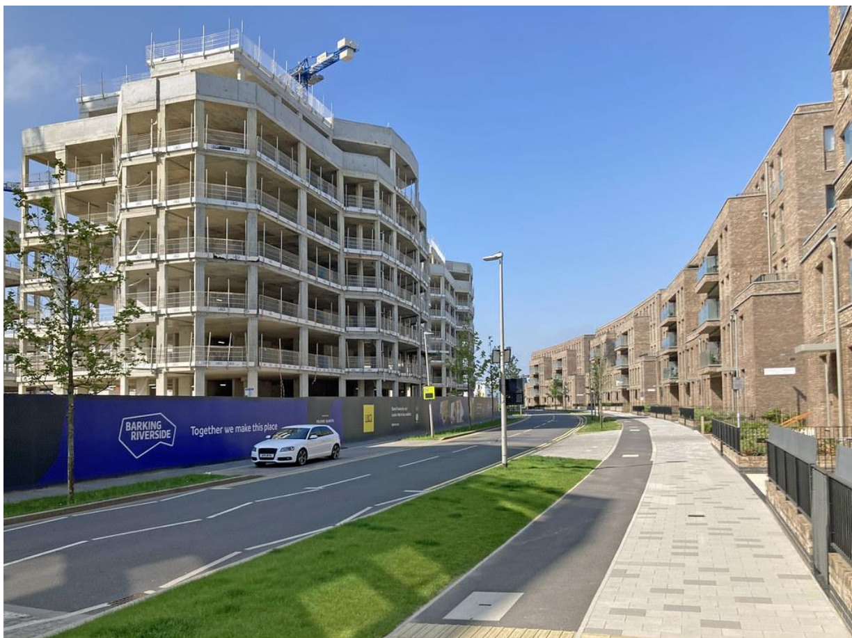
-new flats built in Barking Riverside
